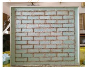
Figure 3: Laid blocks with mortar
