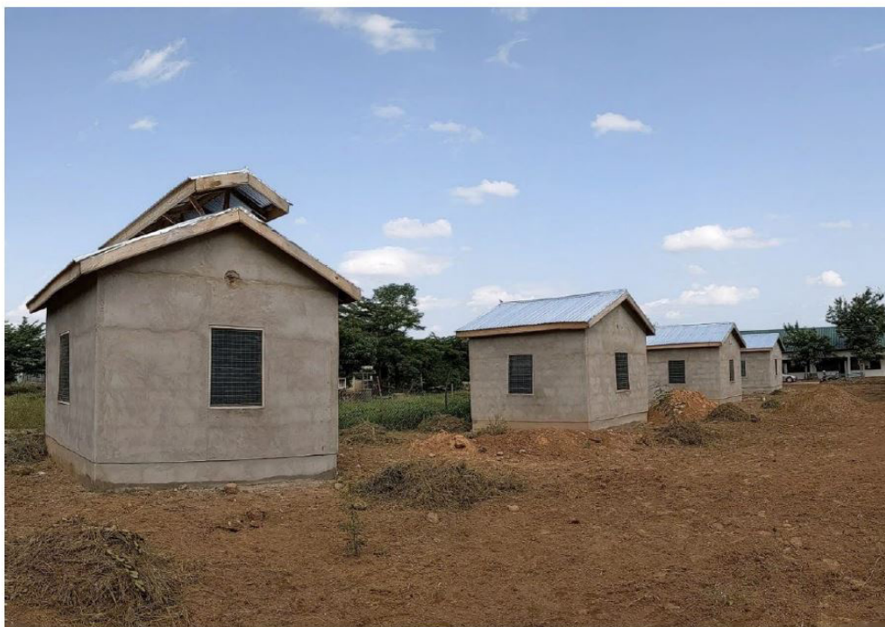
Figure 1: The four experimental buildings (test cells) in Tamale, Ghana. The nearest building has a ridge ventilator.
