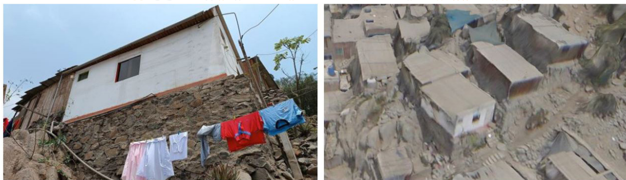
Figure 1: Case study house. Onsite photo (left), 3D reality image from drone survey (right).
