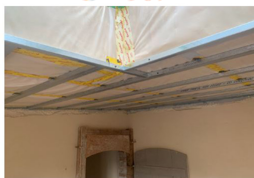
Figure 10: Installation of roof insulation (18 cm mineral wool)
