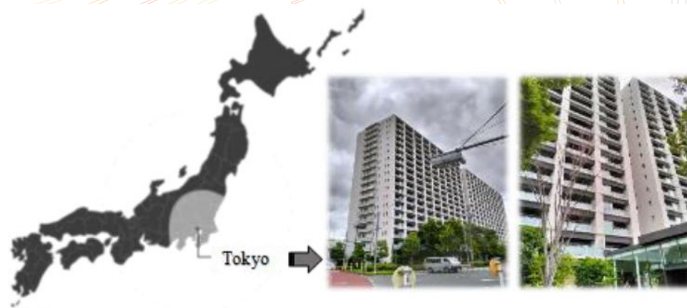
Figure 2: Field measurement location and targeted building. (Source: Google Map).
