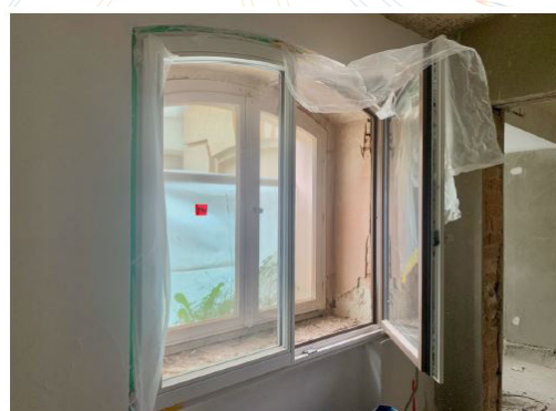
Figure 9: Photo of window enhancements
