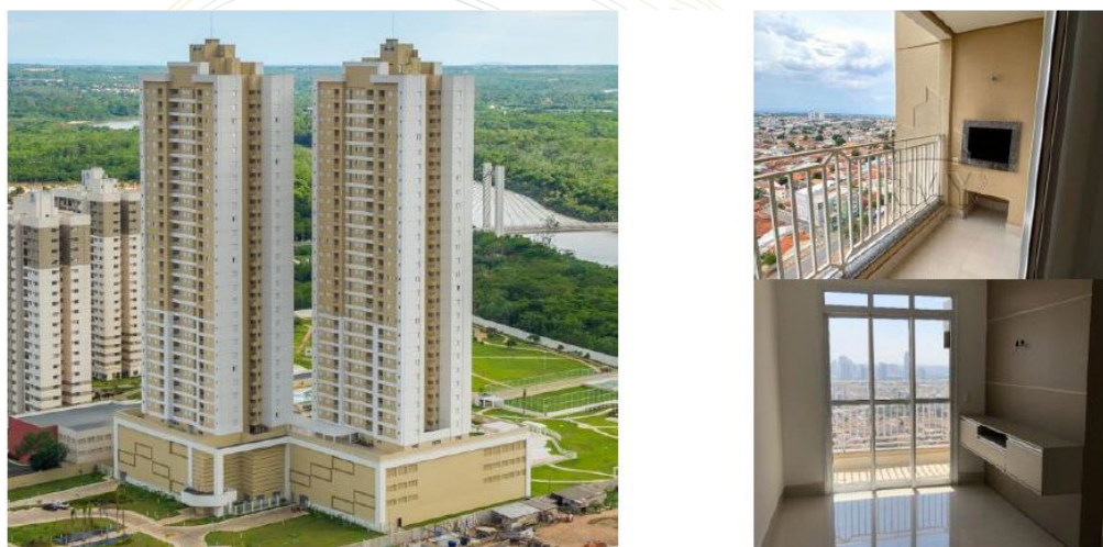
Figure 1: Residential towers Jardim Beira Rio, Cuiabá – MT – Building external perspective, balcony and living room.
